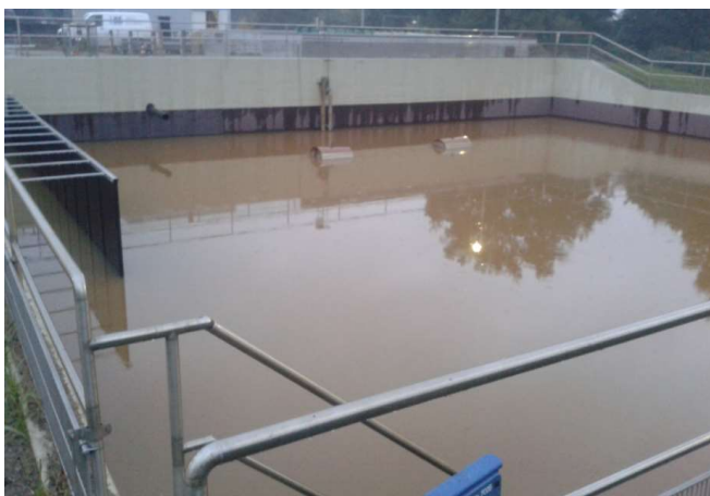
Before OLOID installation
